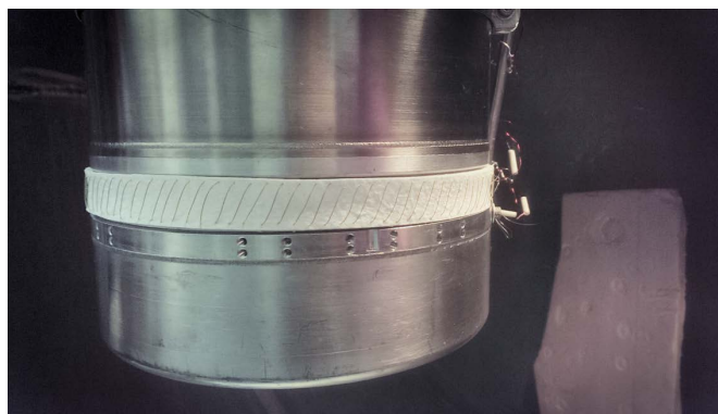
Figure 4.9: Photograph of the D 2 electric heater partially installed.
